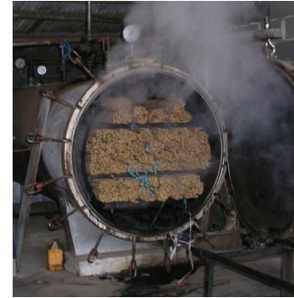
Steam treatment autoclave
